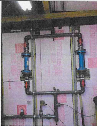
KMnO4 injection point, followed by 2 static mixers
