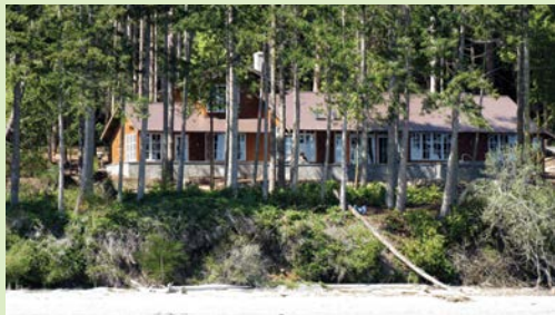
New construction was set back for long-term safety.
